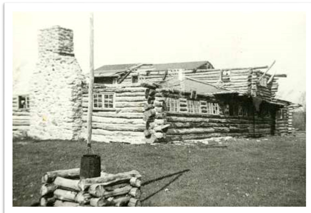
Above: Liberty Hill Log Cabin showing damage from 1938 hurricane, with upper portion of restaurant and chimney top missing. Photo taken September 21, 1938.
