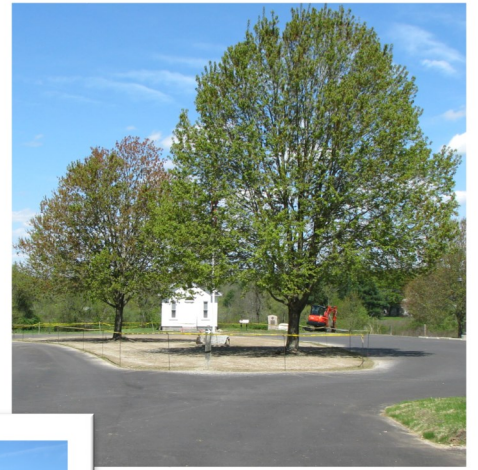
Improvements to our “little green” and driveway
