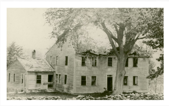
1890 photo of the Masonic Lodge with caved-in roof
